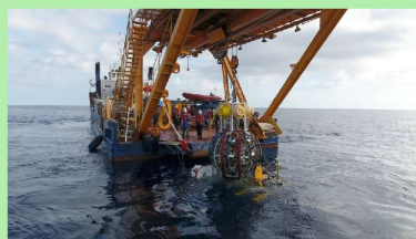
Installation of the 1 st ORCA DU
