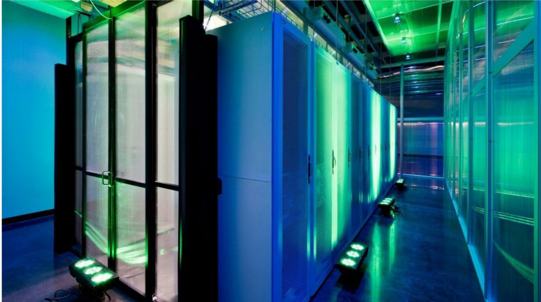
Figure 6: Google's hot aisle containment configuration.
